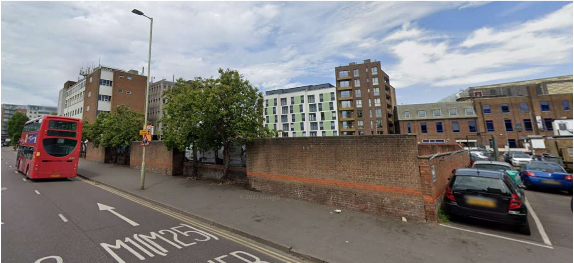
View of the site from Exchange Road looking towards the front elevations of The Clock House and 60 High Street.
