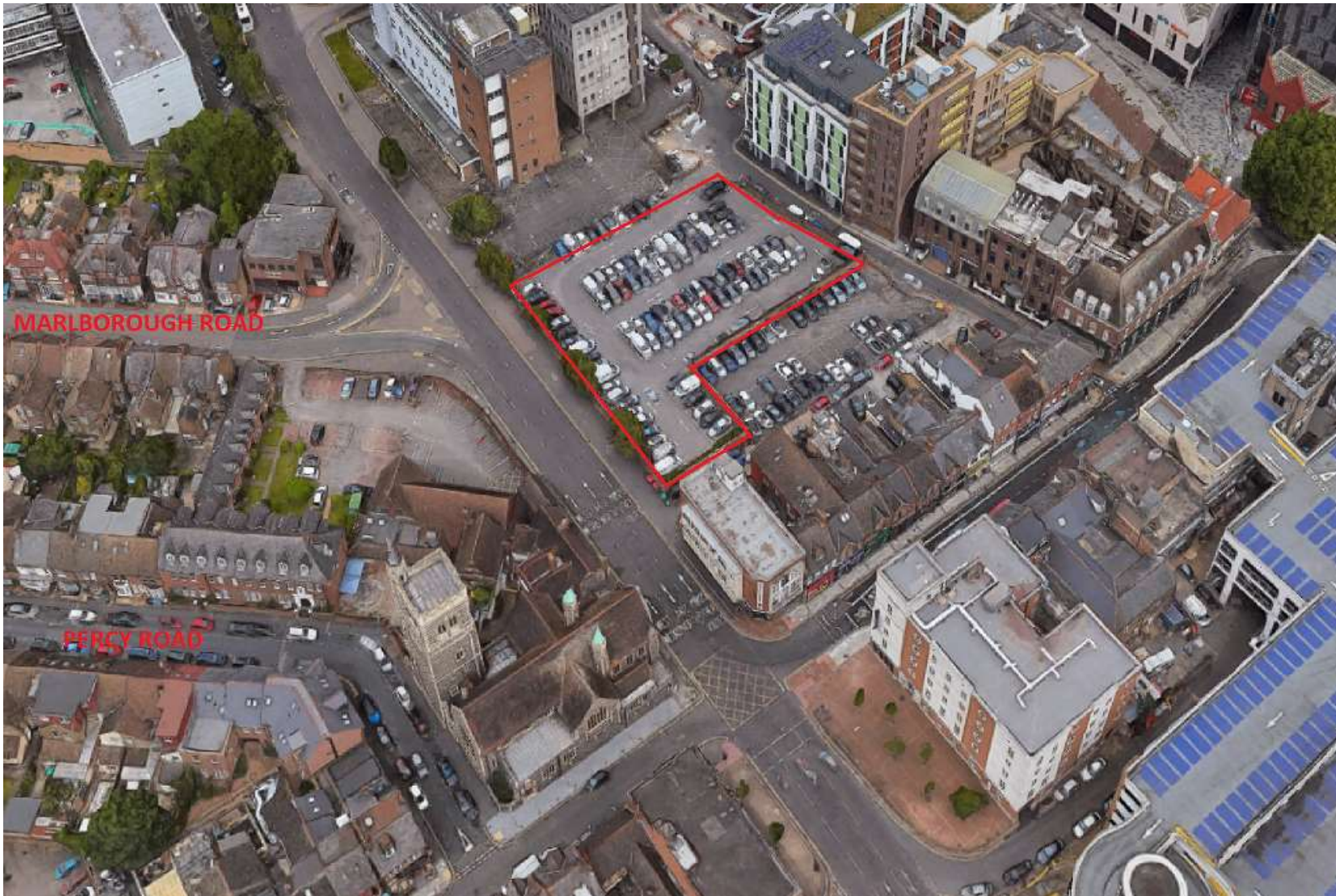
Aerial view of the site and surroundings
